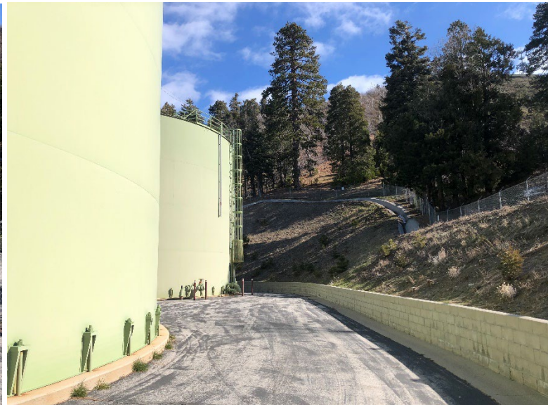
Figure 1 - 2 tanks SCADA and Data Collector
