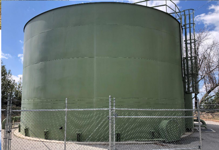
Figure 7 – Beacon I & II
