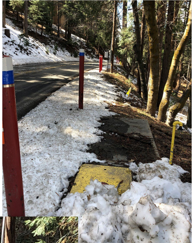
Figure 2 - CLAWA intertie, SCADA flow capability
