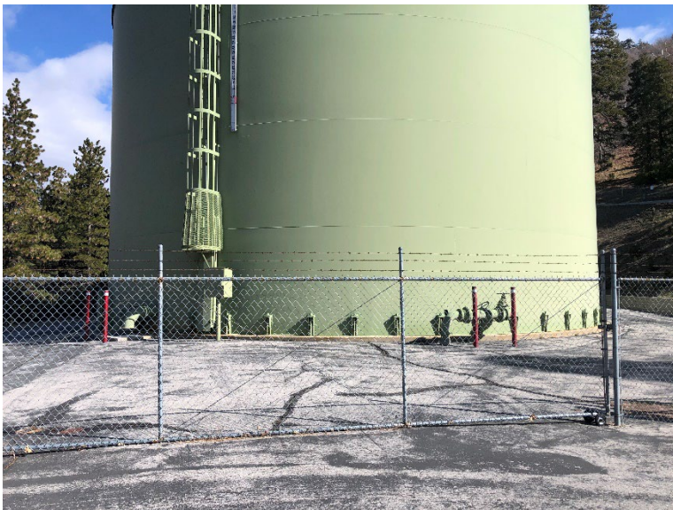
Figure 1 - 2 tanks SCADA and Data Collector
