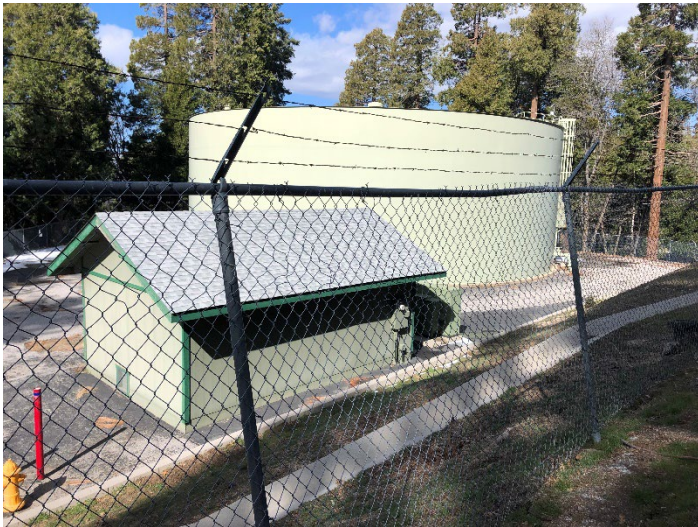
Figure 1 – Chamois Tank Site
