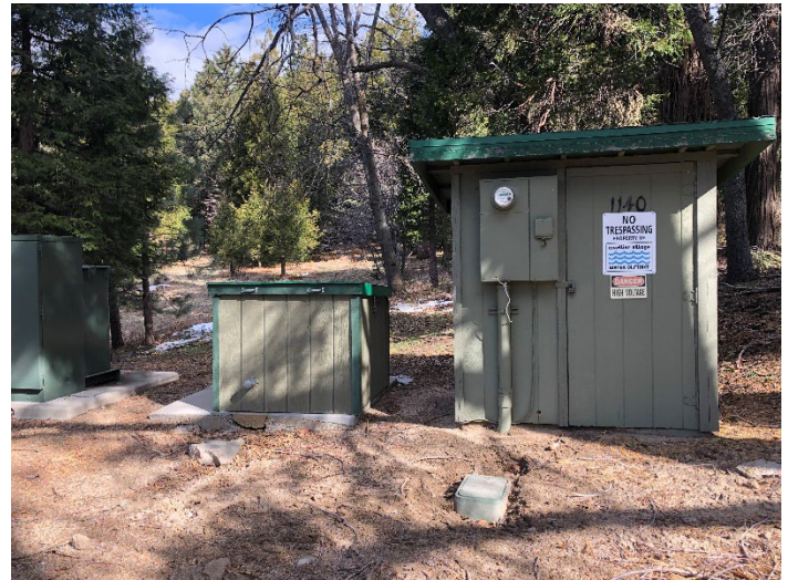
Figure 6 - 1 vertical well – Phosphate injection
