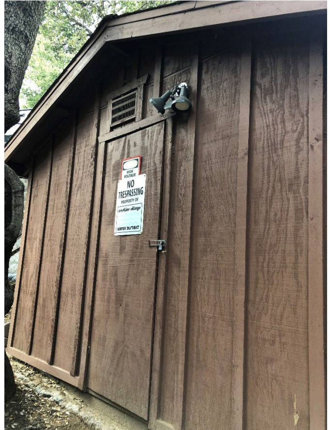
Wabern Pump House – Transfer Only
