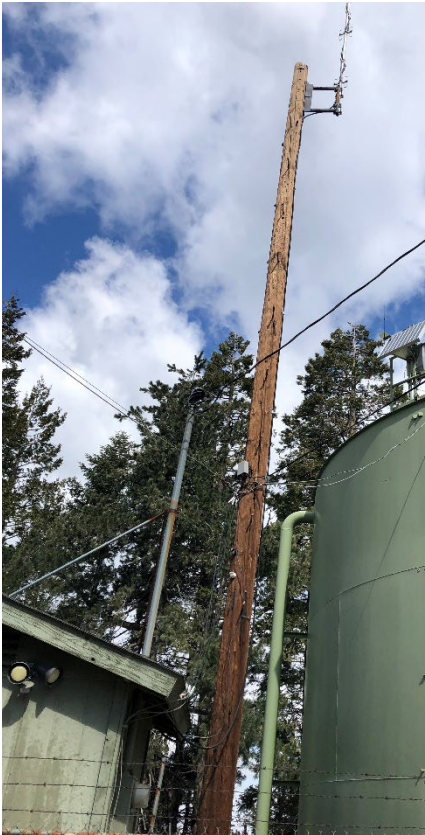
Figure 8 – Beacon I & II
