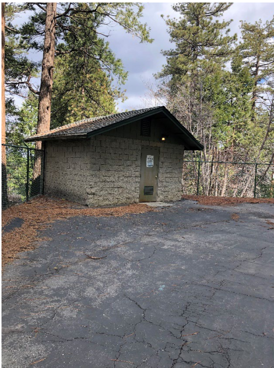
Figure 4 - CLAVAL PRV station (Hydraulically controlled), SCADA and data collection
