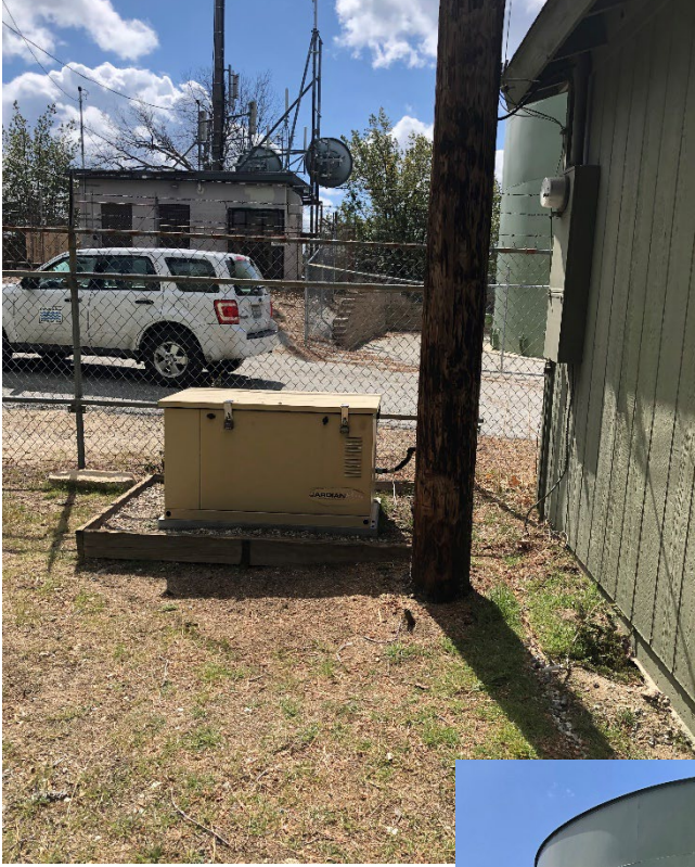
Figure 5 – Beacon I & II
